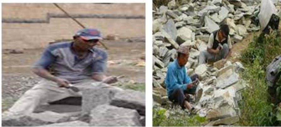
Fig 15(a) Chisel the stone
