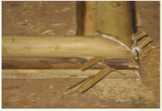
Figure 12 joint with fastener
