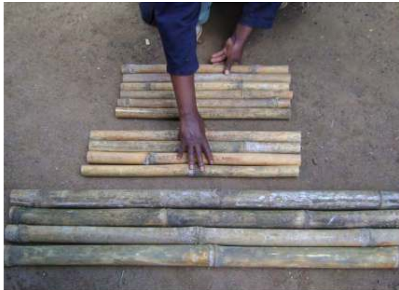
Figure 2 selecting and sorting poles
