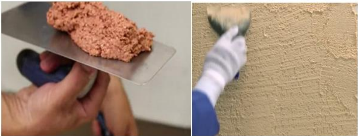
Figure 0-20Apply and Scrap
