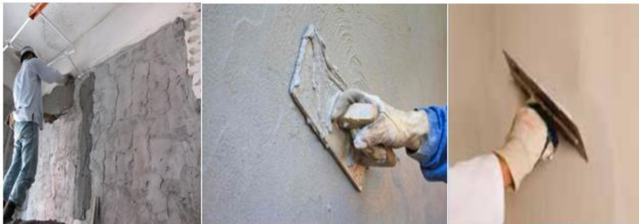
Figure 0-3Applying of Finishing coat of plastering work
