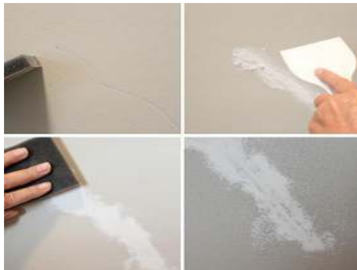
Figure 0-6 Sand the Surface:
