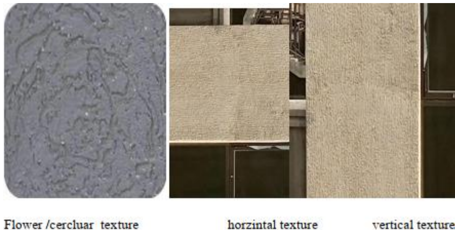
Figure 0-14Circular, Horizontal and Vertical Finish
