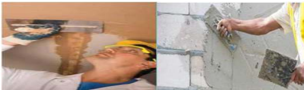
Figure 0-2 Applying of base coat of plastering for brick masonry
