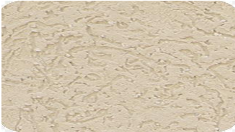
Figure 0-13Circular Finish:
