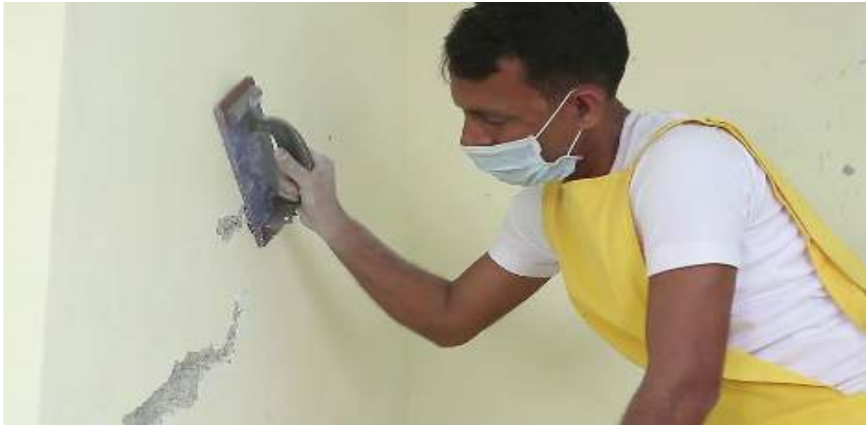
Figure 0-4Clean the Surface
