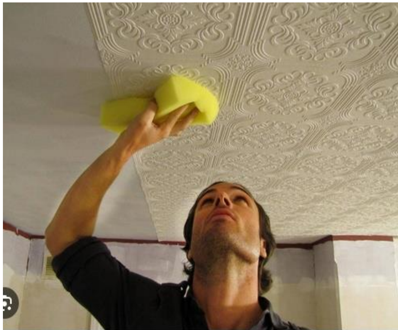
Fig 4.3 Applying match pattern in ceiling
