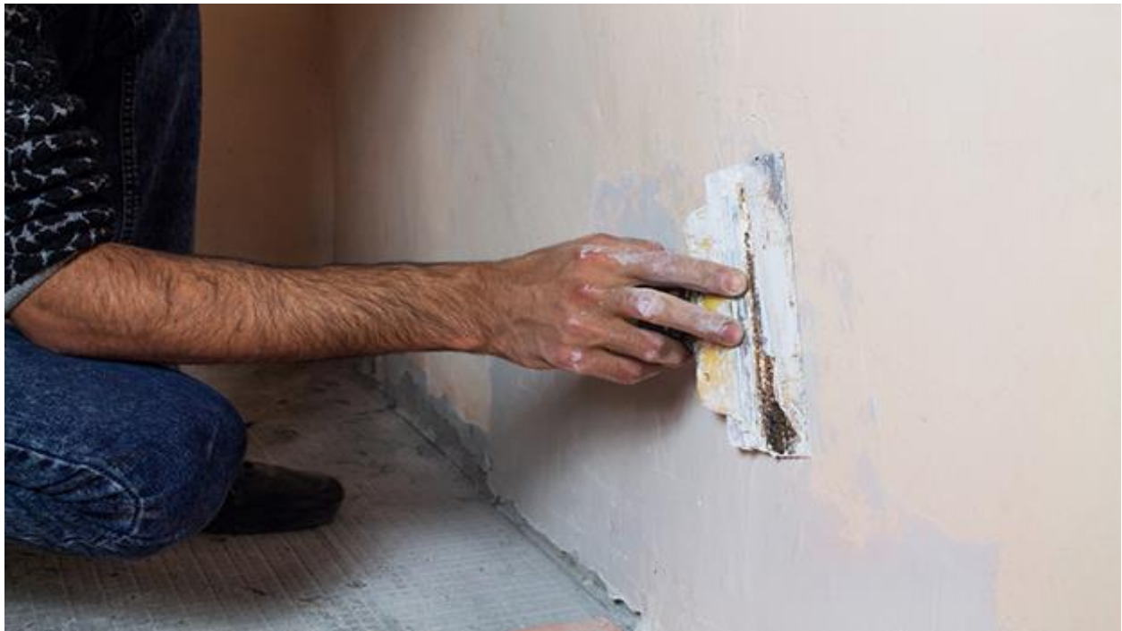
Fig.2.6. Repairing damage wall
