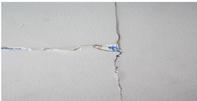
Fig.2.3 Impact of structural movement
