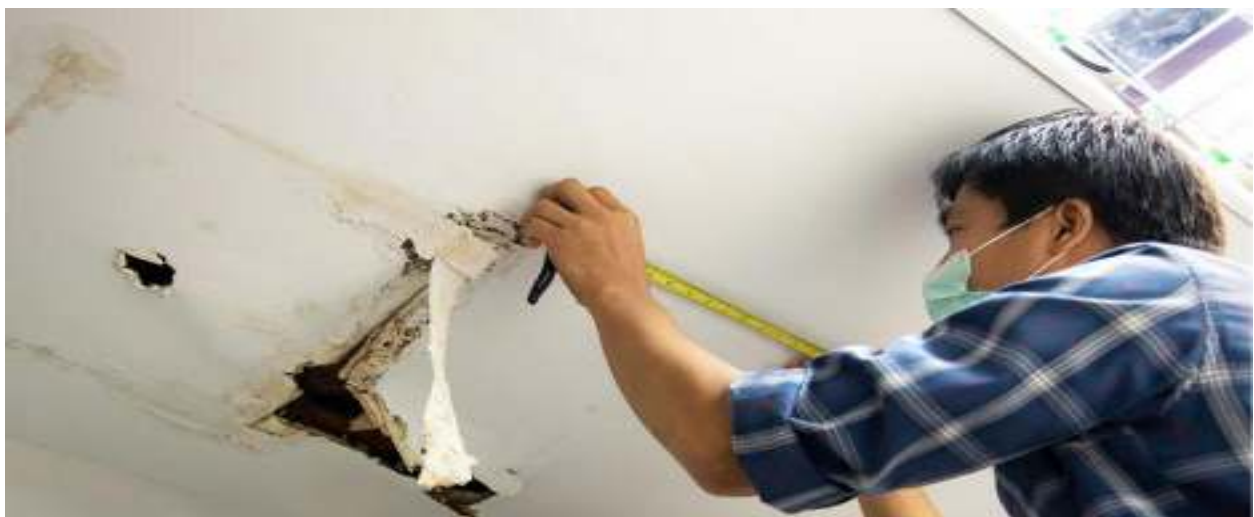
Fig .2.1 moisture and water damage
