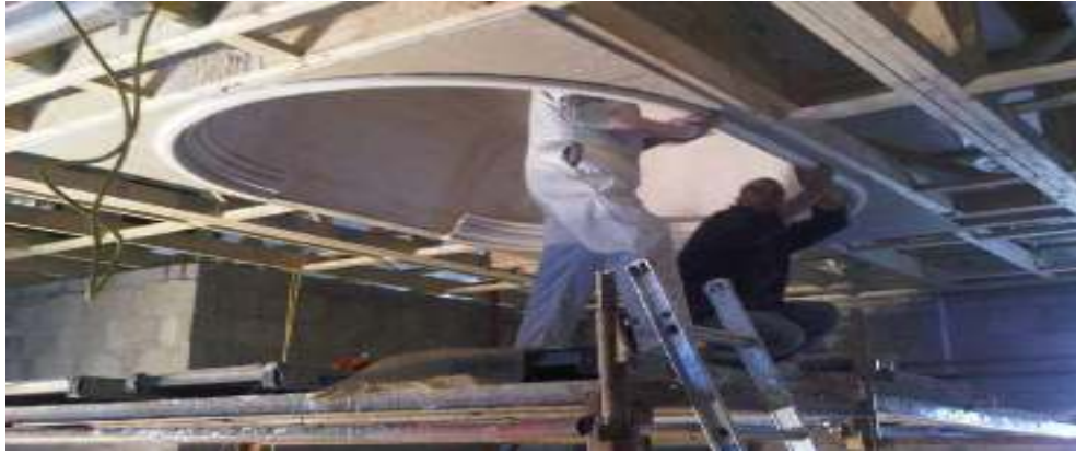
Fig 1.1 fixing fibrous plaster
