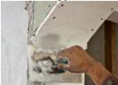
2. Finishing plasterboard
