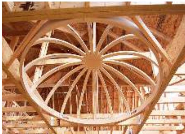
Fig 2.3 Arch timber frame
