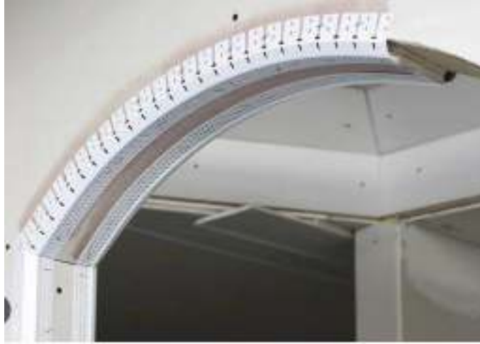
Fig 5.3 Paper-Faced Metal Arch Beading:
