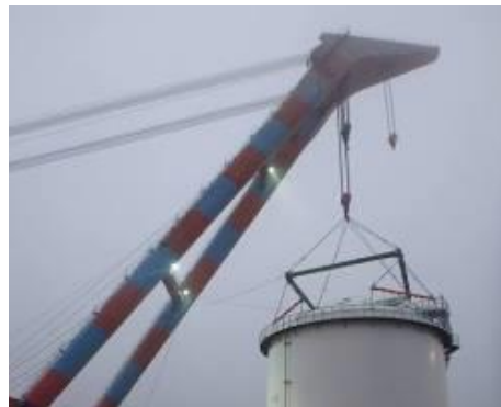
Figure 3.7 Rigging and hoisting a storage tank
