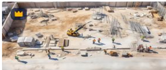
Fig. 2.1 facility arranged work site
