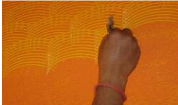
Fig 3.7 Combing or Dragging:
