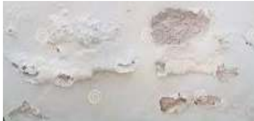
Fig 3.16 Efflorescence
