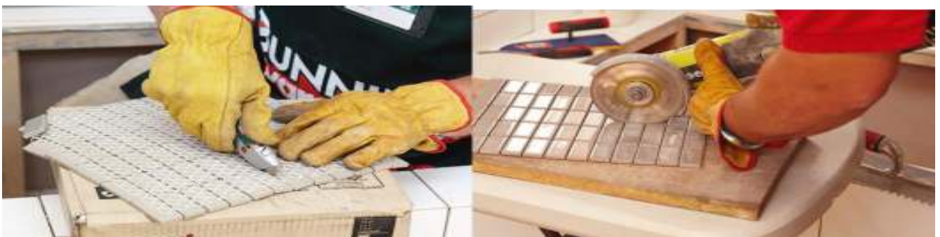
Figure 4-4cutting mosaic tiles for walls and floors
