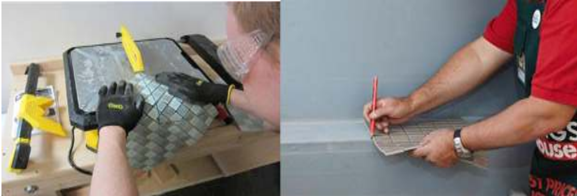
Figure 4-3 Cutting and shaping tiles
