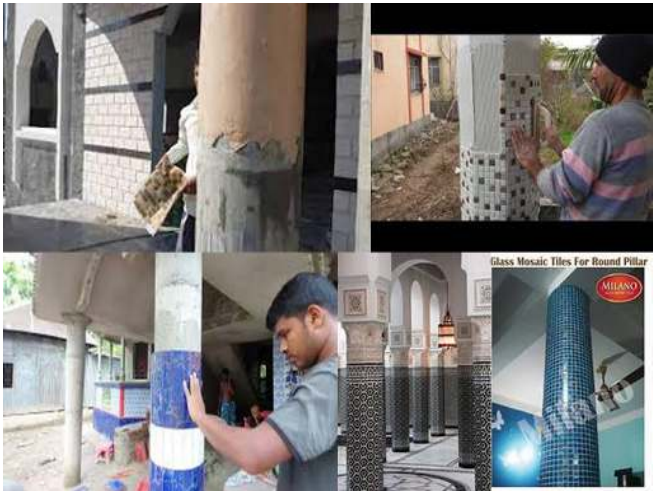
Figure 4-11 fixing decorative mosaic tiles on a circular column
