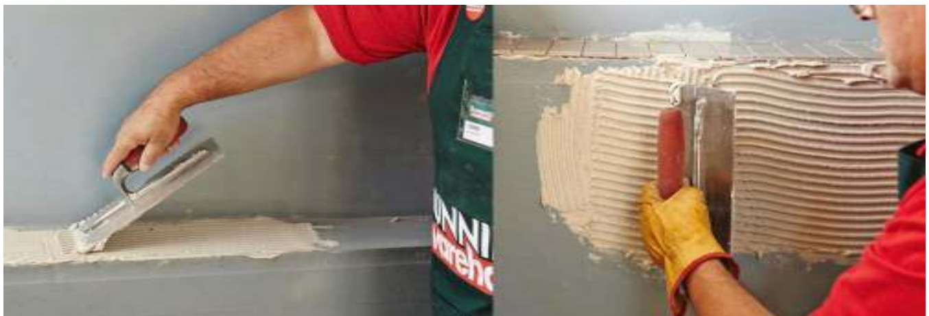
Figure 4-7 applying mortar and/or adhesive on the wall
