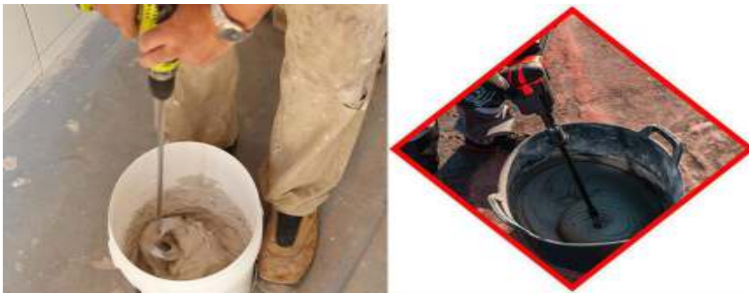
Figure 4-0-6 Mix mortar and/or adhesive
